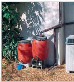
Gutters and downspouts funnel rainwater to the rain barrels.
