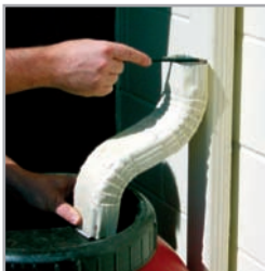
Mark downspout for cutting
