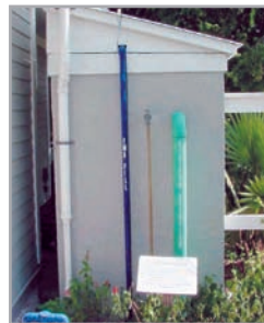
These cisterns at the Florida House Learning Center each hold 2,500 gallons of rainwater.
