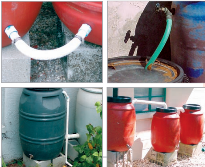
Types of connections: flexible hose clamped on PVC fittings (top left), garden hose (top right), 2" PVC pipe connected at bottom of barrels (bottom left), 2" PVC pipe connected at top of barrels (bottom right).
